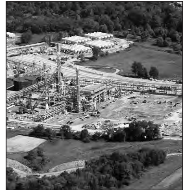
Fracking in eastern Ohio. Photo by Ted Auch, FracTracker.
